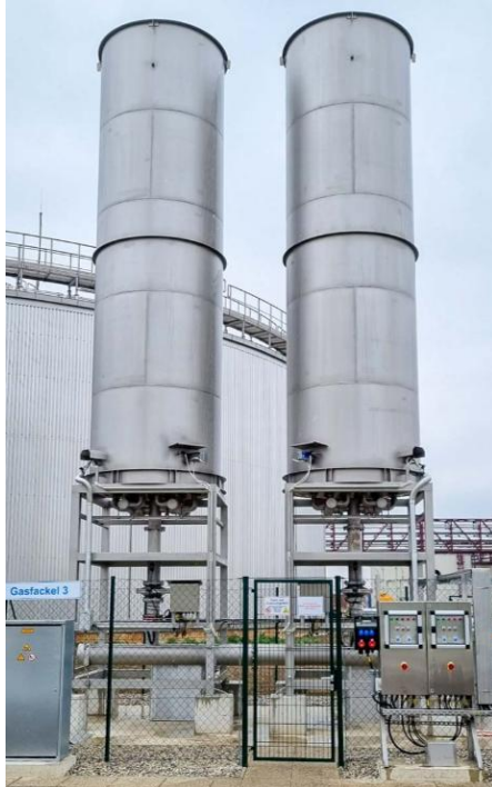
Figure 2-6 Typical Enclosed Flare (Himmel)
