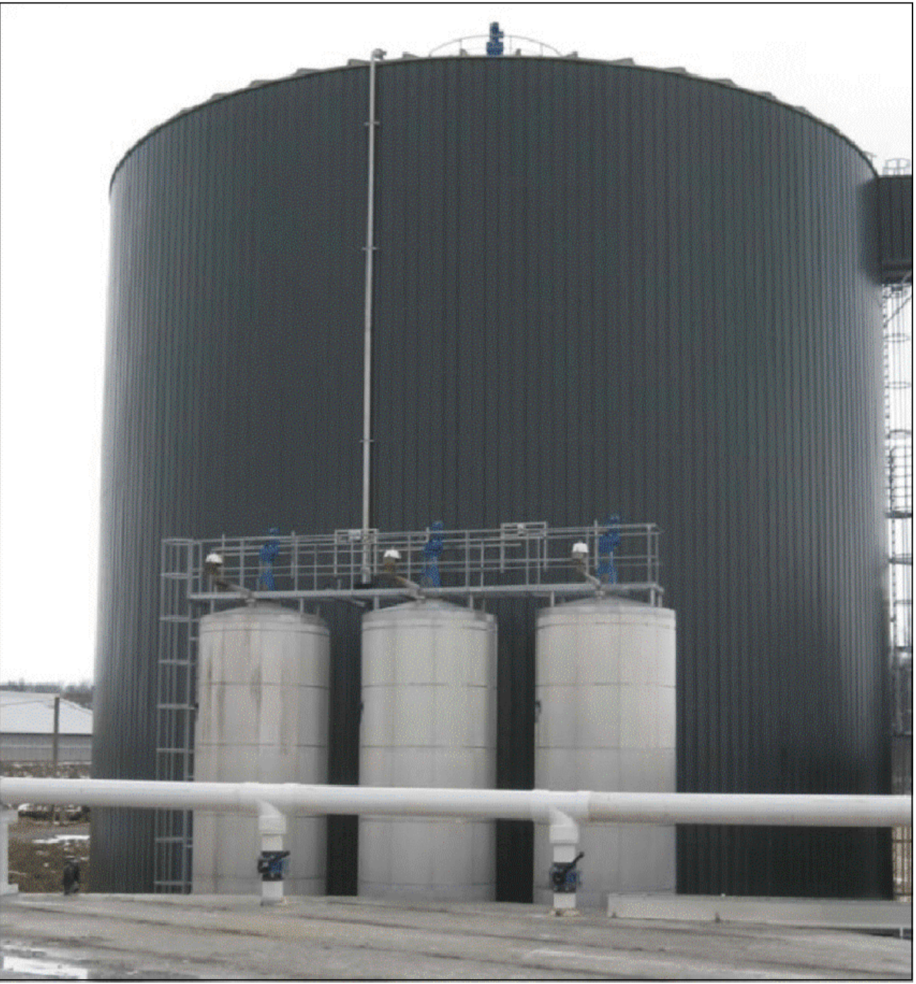
TYPICAL PASTEURISATION TANKS (N.T.S.) (FOREGROUND)
