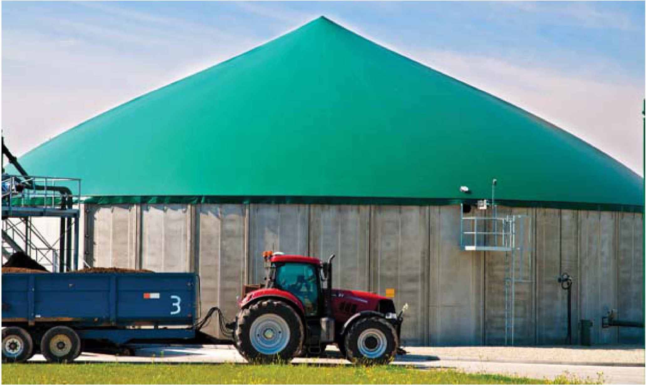
POST DIGESTION DIGESTATE STORAGE TANK (N.T.S)
